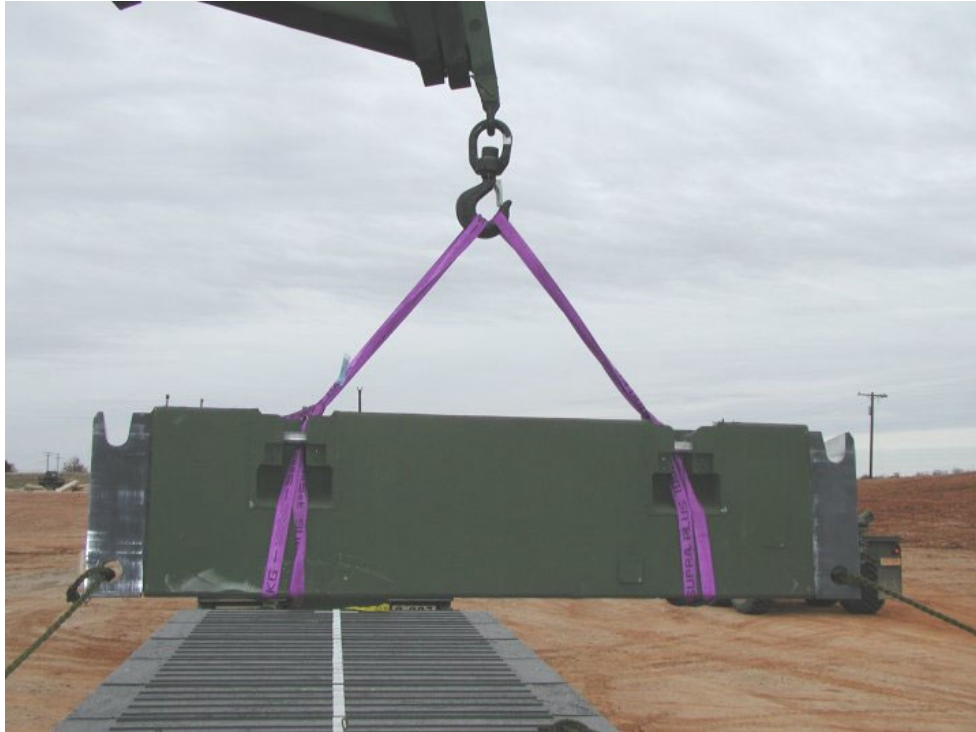
End Beam Slings Positioned
