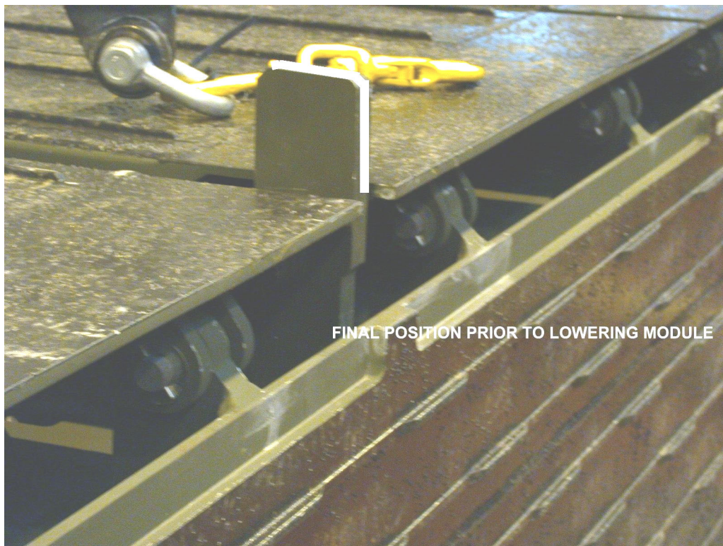
Figure 11. 100 Transport Aid Inserted Under Deck Unit
